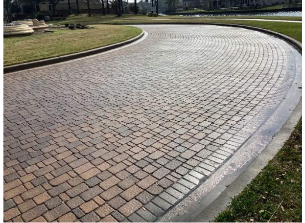
Pavers overview at main entrance
