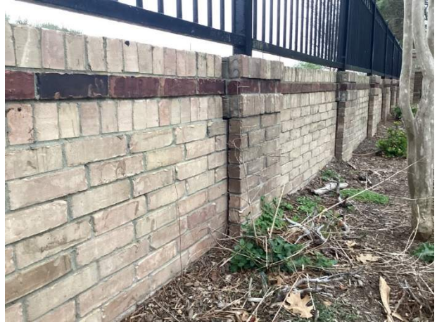
Panelized masonry perimeter wall under fencing
