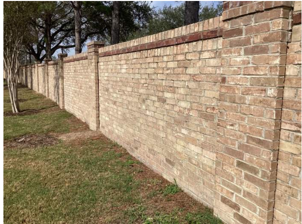
Panelized masonry perimeter wall overview at the manors
