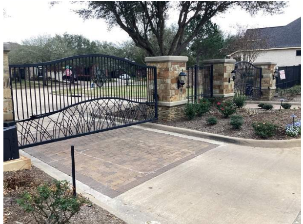
Steel gates at the villas
