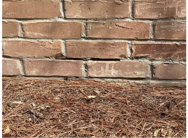
Wall exposed support wire
