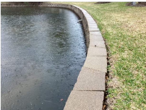
Masonry retaining wall
