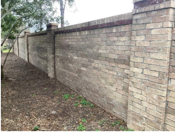
Panelized masonry perimeter wall overview
