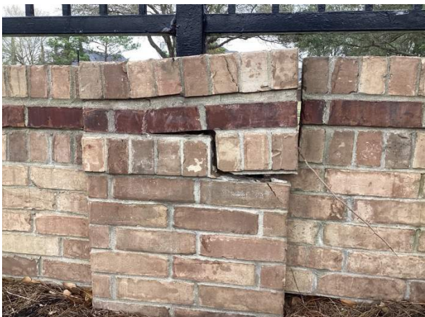
Wall displacement
